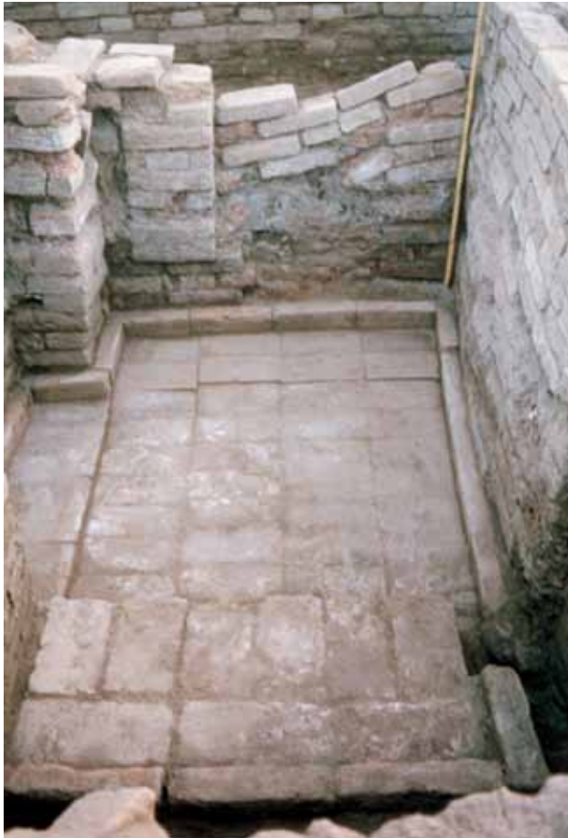
A bath floor in house with outlet to street drain
